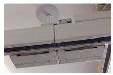
Our unique gate system fitted to ensure the tracking is correctly lined up when transferring between multiple rooms and pieces of ceiling track
