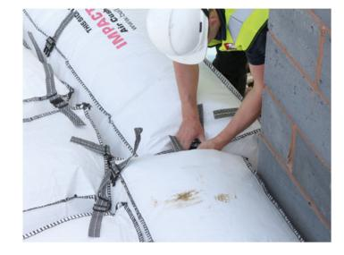
5 Perform a push and fill test and if the bags spread install more bags to reduce any gaps. Push bags up to make room for additional bags. This ensures extra protection.
