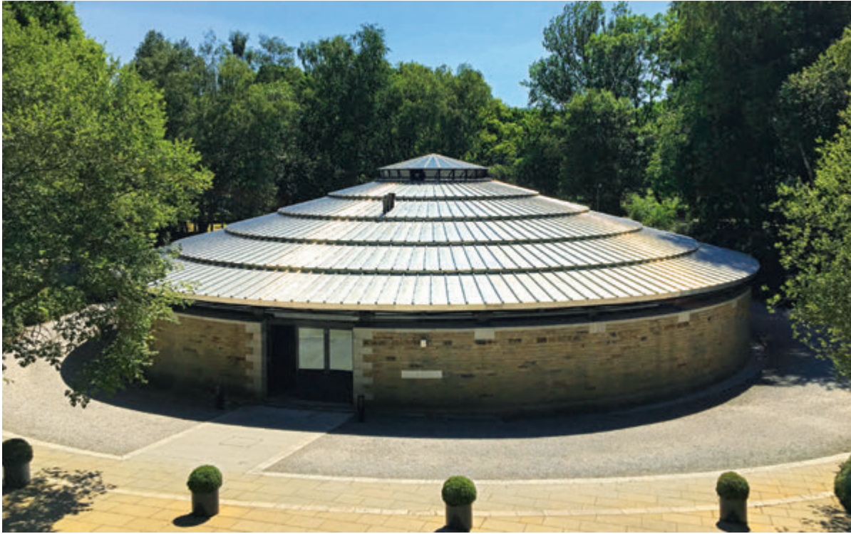
The Round Building Factory
