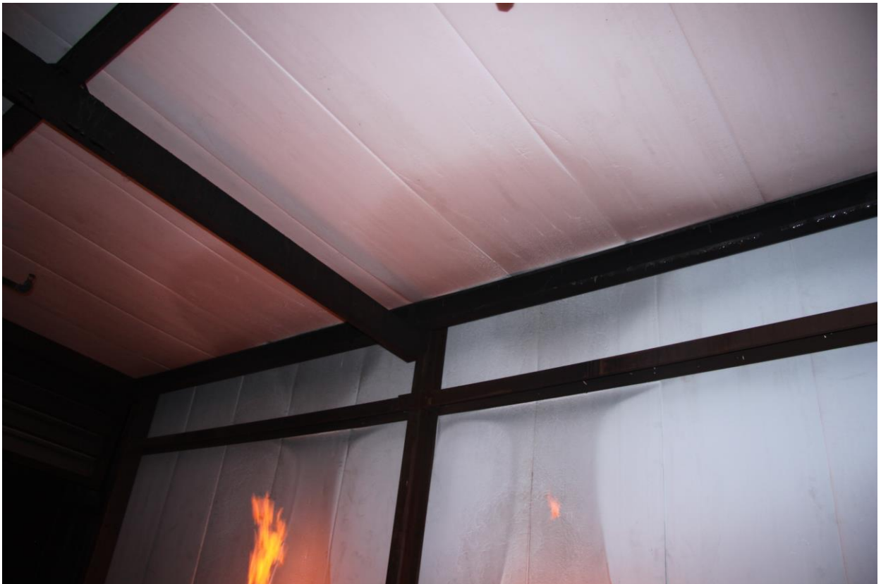
Figure 4.4.6: Heat damage visible on horizontally installed material
