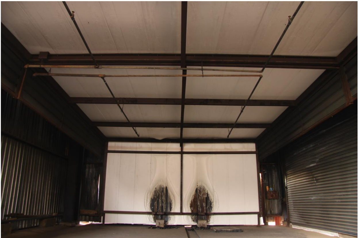
Figure 4.4.8: Test installation after the SANS 10177-11 (V) test was concluded
