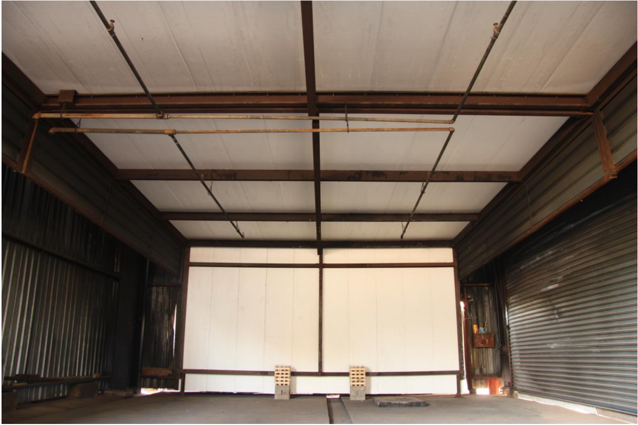
Figure 4.4.1: Test installation prior to ignition of the two Fire Source cribs
