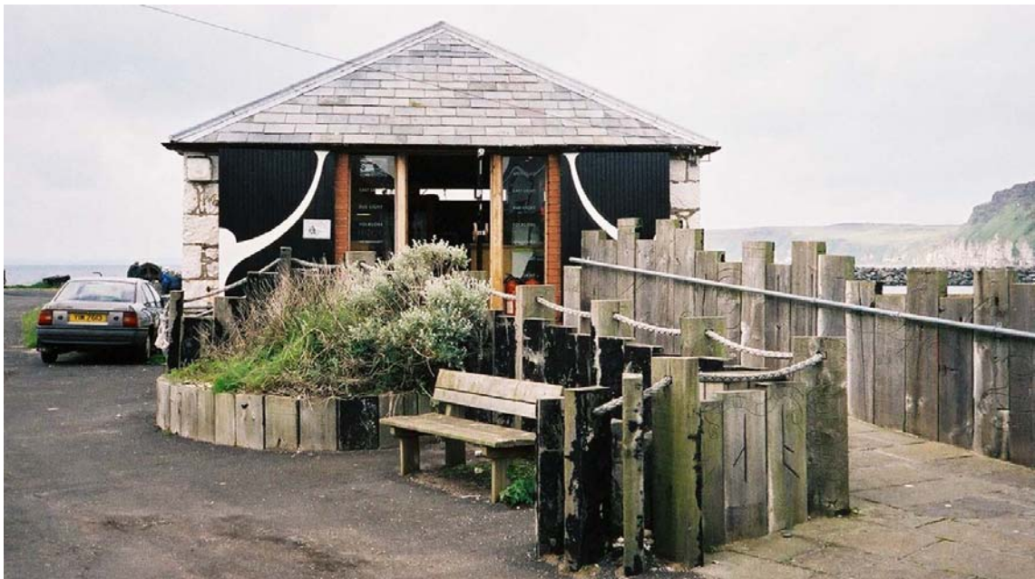
Figure 5.4.1: Rathlin's Boathouse Visitor Centre
