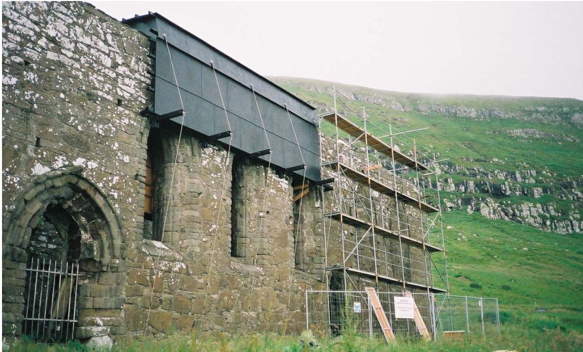
Figure 5.4.2: St Magnus Cathedral, Kirkjubøur, the Faroes (The covering protects the stonework from the wind and rain so that it can dry out to be properly restored.)
