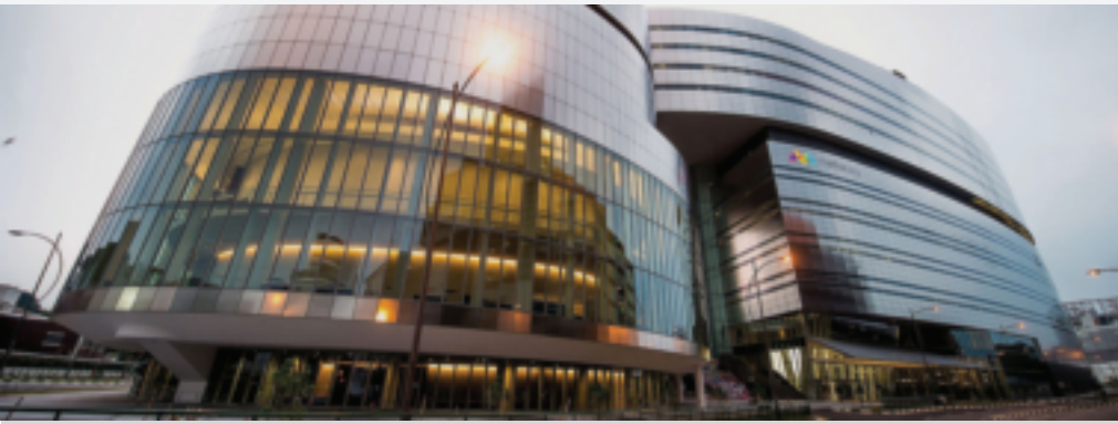
As Mediacorp's consultant and master systems integrator, Qvest Media was commissioned with the overall technological advisory, design and the entire systems integration of the Mediacorp Campus, a new 79,500sqm broadcasting and media centre in Singapore.
