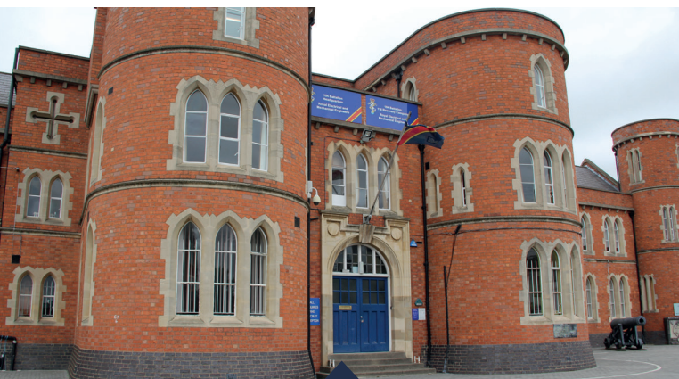
Clare Street Army Reserve Centre.
