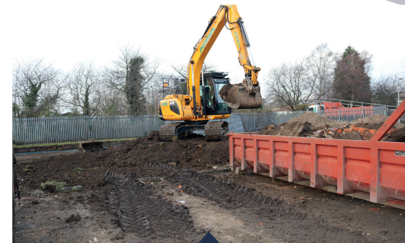
Starting to build a new cadet centre in Derby.
