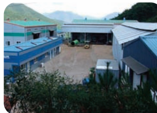
TSA Coating Factory
