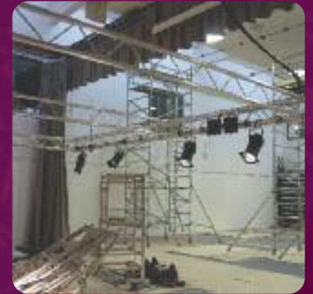
Beckfoot School under construction
