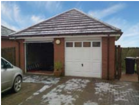
Two 7'0" wide up and over doors too narrow to allow a larger car to get into the garage
