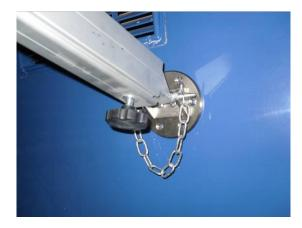
Storm bars that can also be fitted now or when the frame is built are; from the intermediate leg to the next roof rail and also from the corner post to the roof rail. (Refer to plan) These bars are to stabilise the awning and stop the legs from kicking in high winds.
