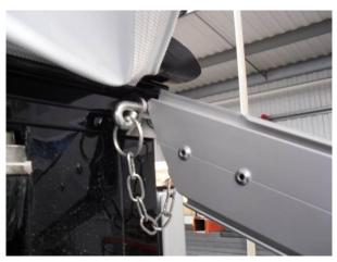
The roof rail is now allowed to slope down and rest on the floor. This operation is now repeated for the remaining roof rails along the main structure.
