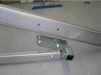
The roof rail is connected to corner post and secured using the 17mm spanners, This assembly is carried out with the parts still on the floor, repeat for each post.
