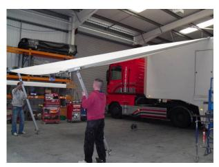
It is recommended that fixing pegs are used to anchor the corner posts into position. The two corners of the front frame should now be tethered to the ground, to help keep the frame in position. This will also stop the roof panels from lifting the frame in windy conditions.
