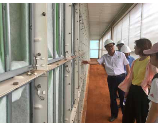
The air purifier provides clean, fresh airflow to the farms and helps reduce pathogen load.
