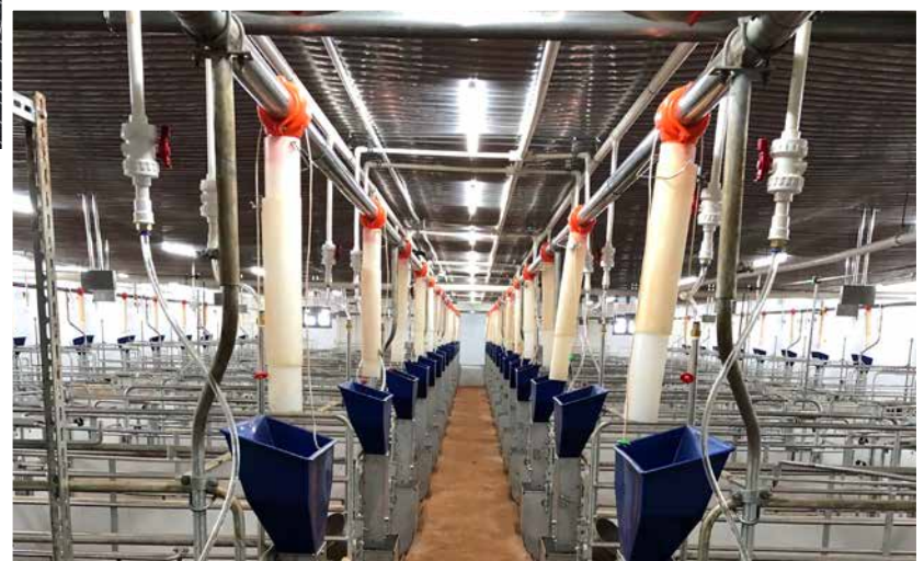
Below: The smaller alley and lower ceiling in pig houses can lead to savings in energy and production costs.
