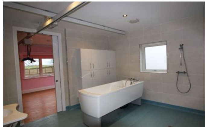
Ensuite bathroom features flexible H frame ceiling tracking with the OT200 ceiling hoist with automatic recharging and emergency lowering function.
