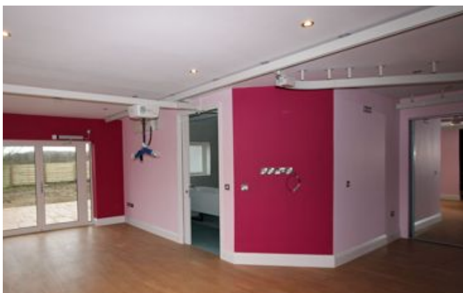
The infra-red, easy glide H systems and 6 hook spreader bars give total flexibility on sling use whether used with walking harnesses for therapy, bathing or simple user transfer
