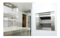
The service lifts we supply are split into two categories – dumbwaiter lifts and trolley lifts. Our Dumbwaiter lifts are small lifts within self-supporting structures that are predominantly used to carry food, drink and kitchen utensils between floors up to 15 metres. These are suitable for both residential and commercial/leisure applications.
