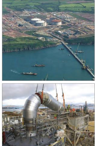
Ledwood have constructed a number of major mechanical constructions. This involved fabricating and delivering prefabricated modules to site with follow on erection and pre-commissioning. The work included detail design of steelwork, heavy lift management and shipping of modules by sea from workshops to site.
