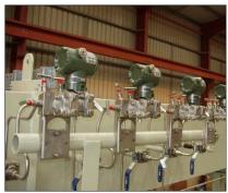
Engineered solutions based on nationally and internationally recognised standards for instrumentation in process control systems
