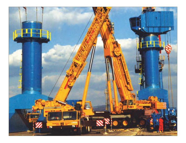
Ledwood has the facilities and expertise to fabricate a wide range of mechanical equipment. The dockside cranes shown above are typical of the large material handling equipment fabricated for various clients. The cranes were outfitted complete with the slewing ring, control cabin and carriages at the quayside in Pembroke Dock before shipment direct to their final location.
