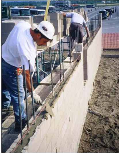
Figure 2-3 Masonry wall under construction (Credit: Masonry Institute of BC).
