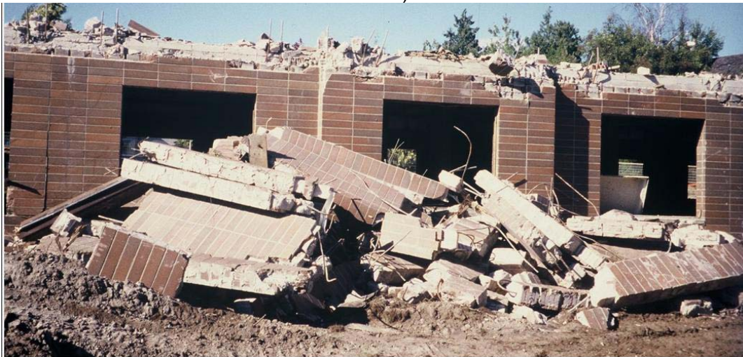
Figure 2-40. Stack pattern walls: a) stack pattern wall in an existing masonry building 1 ; b) demolished stack pattern wall 2 .
