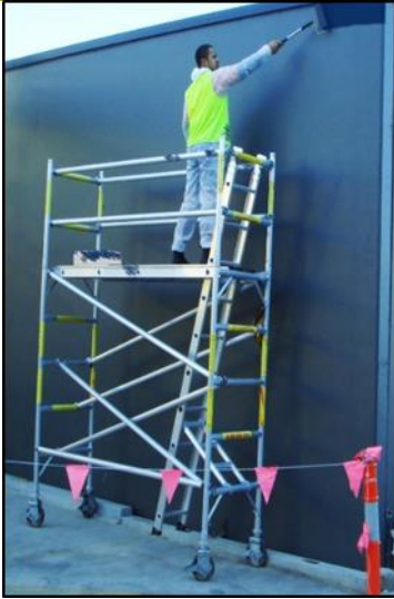
Mobile tower scaffold/double guardrails.
