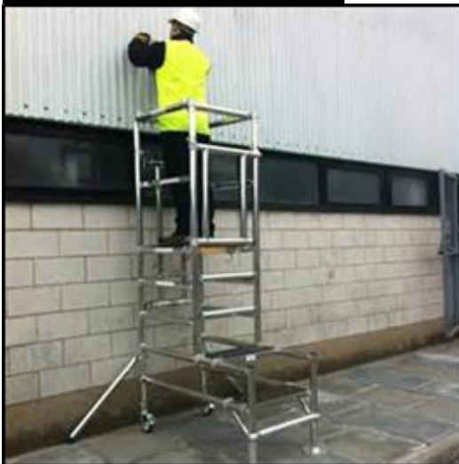
Podium. User protected on all sides by guardrails and cannot fall.
