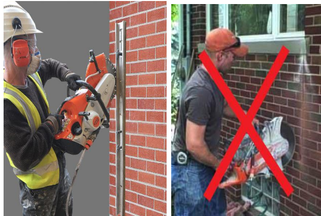
Illustration of controls necessary when cutting silica materials
