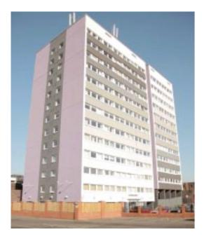
Liscard House, Wirral System: Swisslab EWI Insulation: 60mm Phenolic
