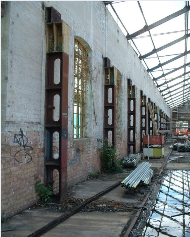
Before: The cast iron columns in 2007 before the blast-cleaning started.
