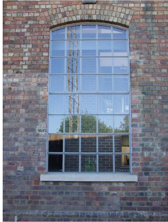
Three frames were cracked and were welded and then blast-cleaned as normal before being coated with Zinga
