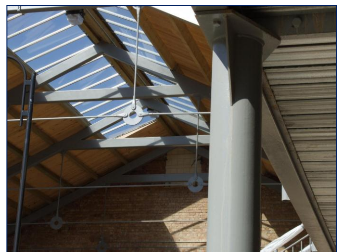
Cast-iron column, wrought iron roof-tie and mild-steel truss
