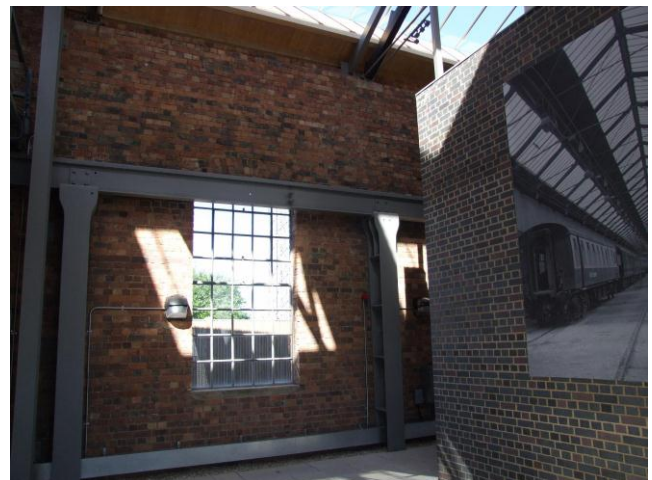
The columns after the new roof has been installed
