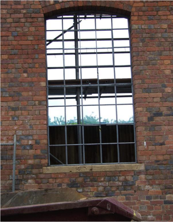
The cast-iron windows measured 5 feet x 12 feet high
