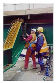
The new cross girders were placed onto the platform by crane at a designated loading position, the platform was then traversed out over the river to the required installation location. The platform was then raised to align the cross girder flange with the longitudinal girder flange and the connection made.
