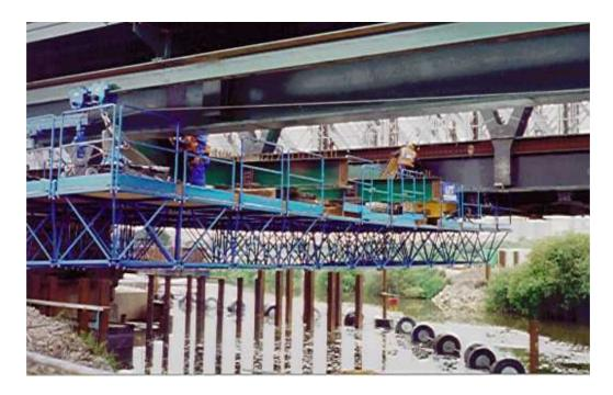
The fully modular Steel 3D Truss Frame platform supplied by ALPS & used during the construction of the Newark Dyke Bow String Rail Bridge had dimensions of 14.64M X 4.88M.
