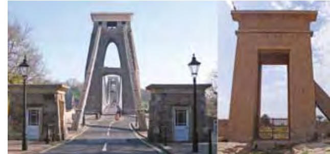
The Clifton Suspension Bridge and one of its prototypes. Photos Dyan Hilton & Aidan Dodson
