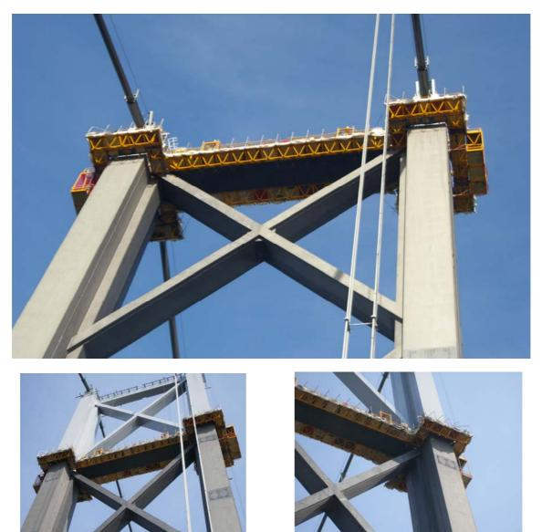
Safety was of paramount importance, the platform being raised and lowered using 12 on board 2400Kg capacity hoists each one protected by a separate independent safety devises. A total of 24 X 100M 16mm wire ropes were used to suspend, raise and lower the platform.
