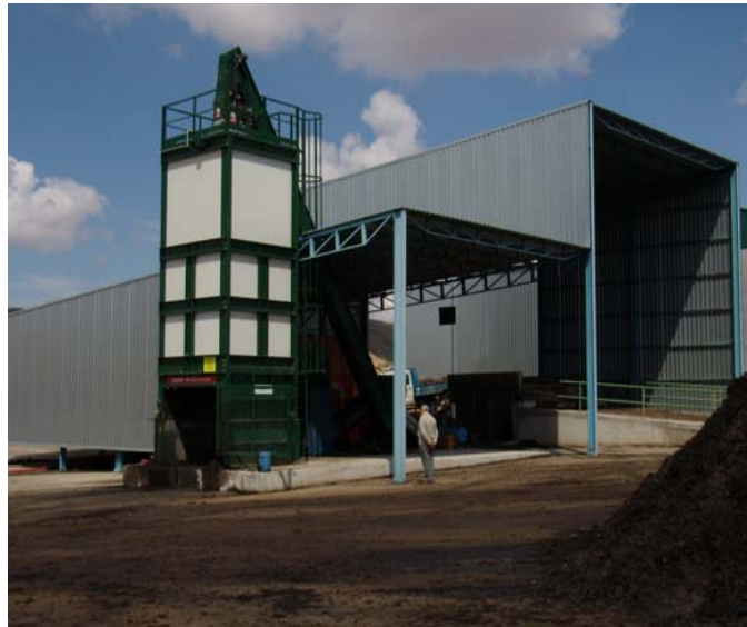
Original VCU system
