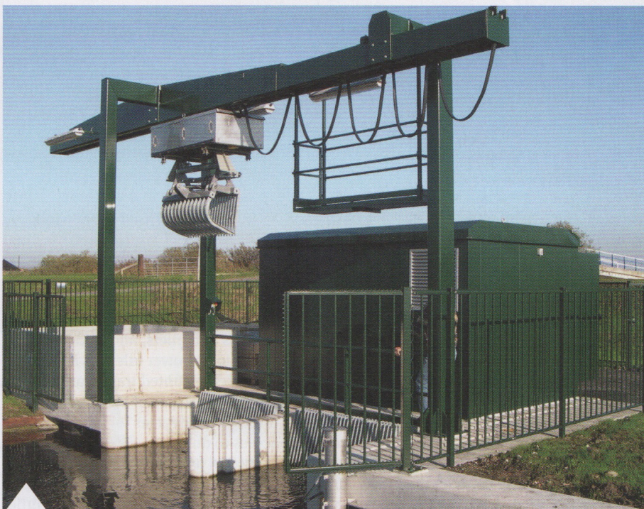
This Bosker trashrake system is an example of pump protection in action
