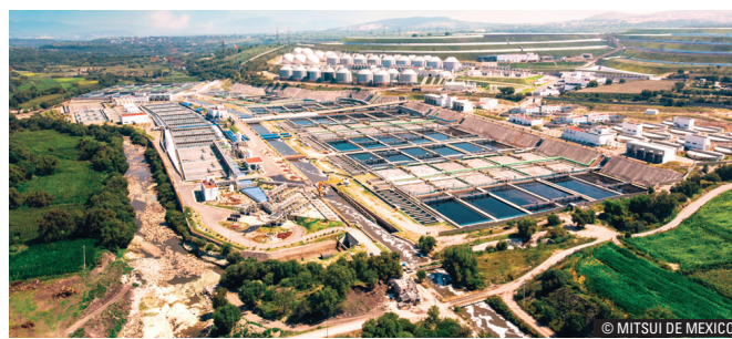
Atonilco water treatment plant
