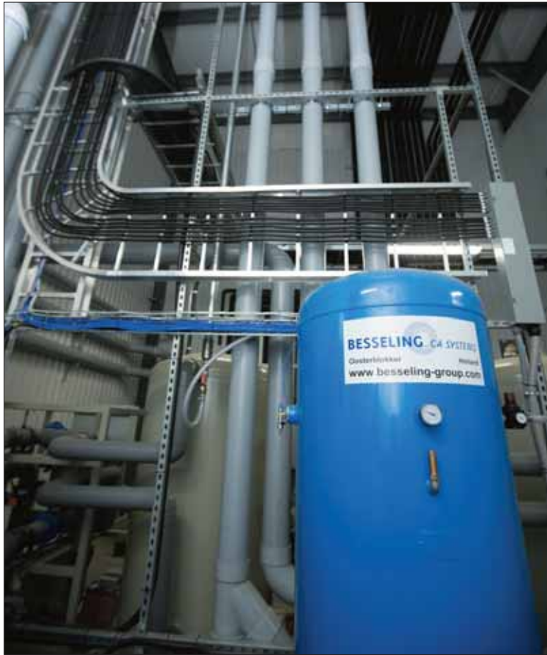
The Dutch expertise of Besseling CA Systems was contracted for the installation of controlled atmosphere rooms, panels and doors.
