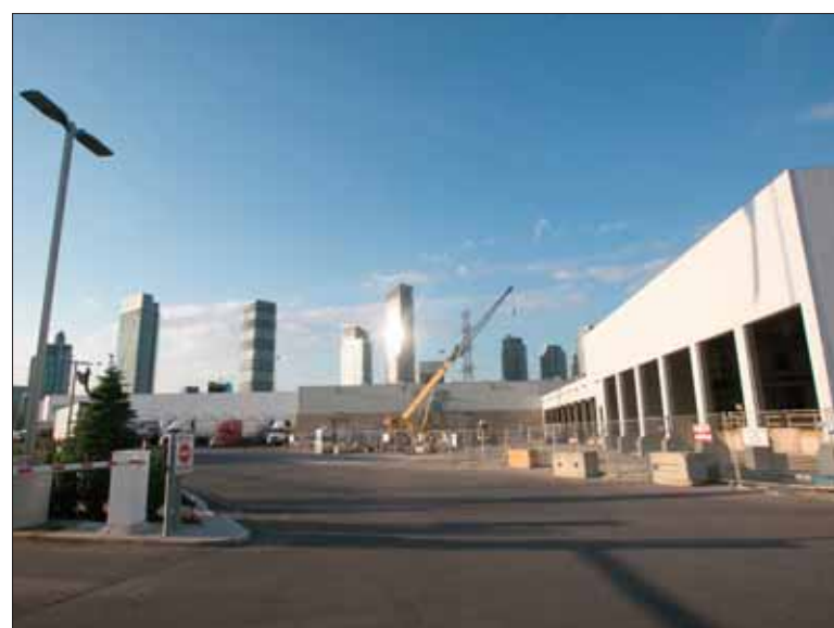
An extension of the southeast loading dock will be finished this month to provide 35 tractor trailer parking spaces for buyers. The 40-foot dock will allow buyers to assemble loads efficiently and safely.
