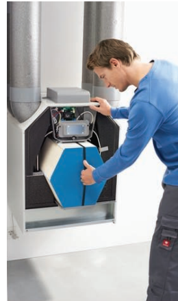
Cleaning the heat exchanger
