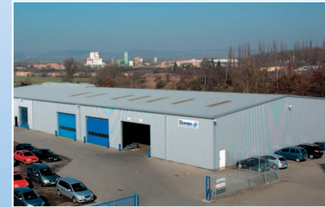
Durwen Production facilities
