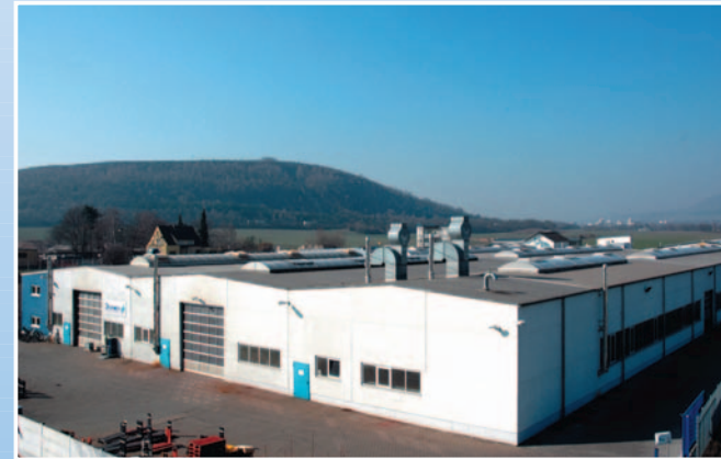
Durwen Production facilities
