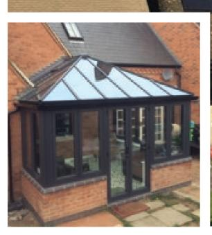
Unlike traditional conservatory roofs which can be cluttered by low hanging bars, oversized ridges and obtrusive ridge ends, and poor thermal efficiency, the Sherborne Roof benefits from a 70% slimmer ridge with the hidden or subtle bars – more glass, less roof and unrivalled thermal efficiency.
