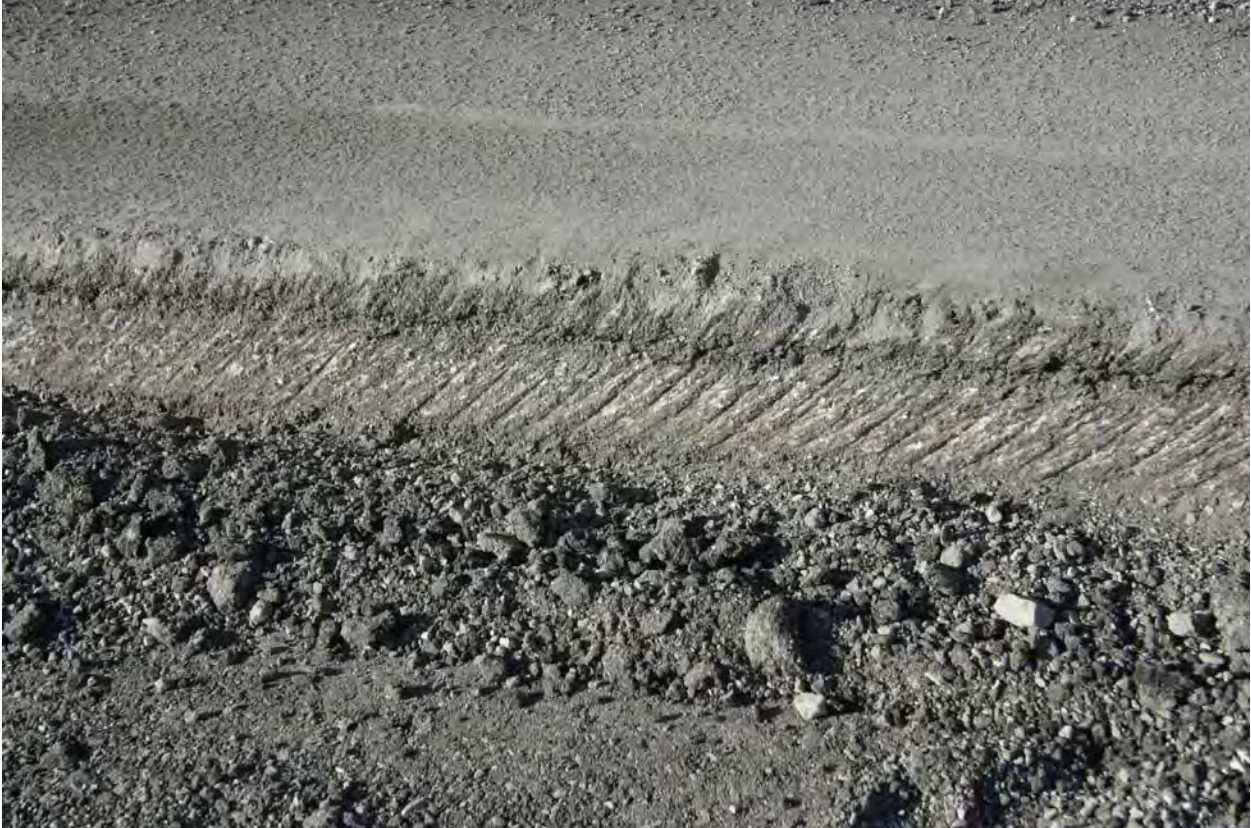
FIGURE 2 Scarified vertical pavement face.
