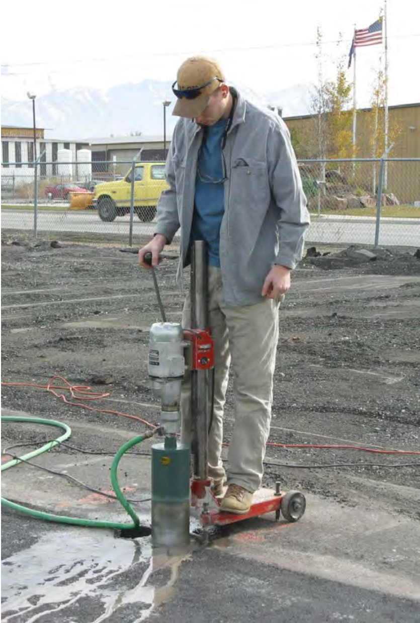
FIGURE 5 Removal of asphalt core specimens.
