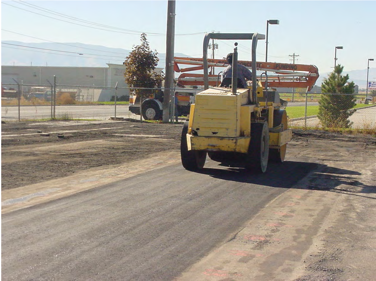
FIGURE 4 Compaction of patch material at test site.
