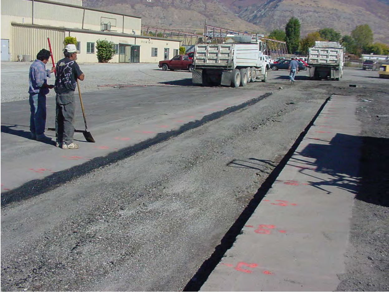
FIGURE 3 Testing site after asphalt removal.
