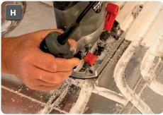
Using a router with bit set to 17mm depth gently cut the new channel following the marker pen layout **(H)**. Ensure the channel is clear and free from debris, if required the channel can be lined with aluminium tape. Lining with aluminium tape is not required in areas with highly concentrated/close floor heating pipes.
