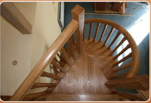
Landings can be supplied to fit round or square holes or as in the stair illustrated "free space" with the landing providing the connection to the upper floor.
