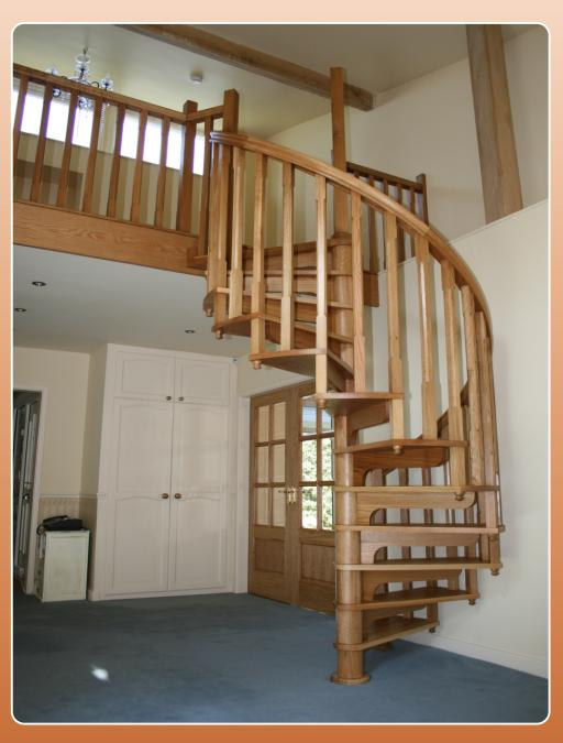
This magnificent hand built spiral staircase is ideal for modern contemporary homes or Barn conversions alike, serving an upper floor, mezzanine or balcony. This image shows clearly the quality of the solid oak treads, balusters and handrail. This stair fully complies with building regulations with no gap greater than 100mm.
