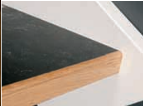
Linoleum covered tread with timber nosing.
