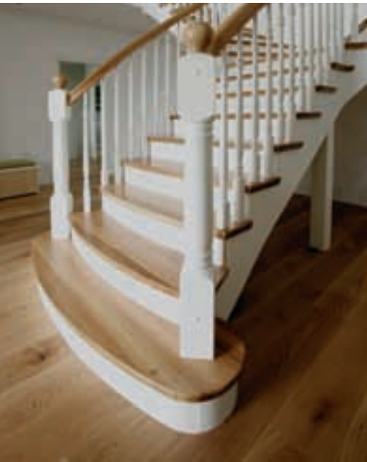
Full bull nose tread with rounded front
