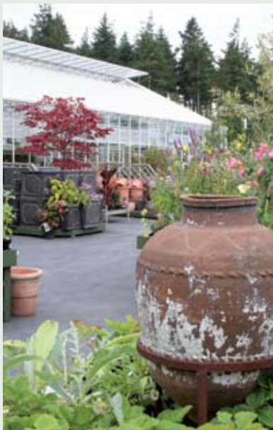
Duchy Nursery - new plant retail greenhouse and courtyard
