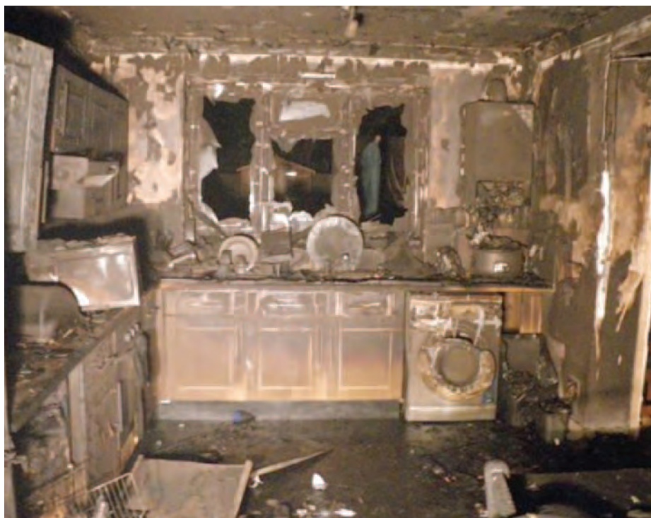
The damage in a home after a tumble dryer caught fire.
