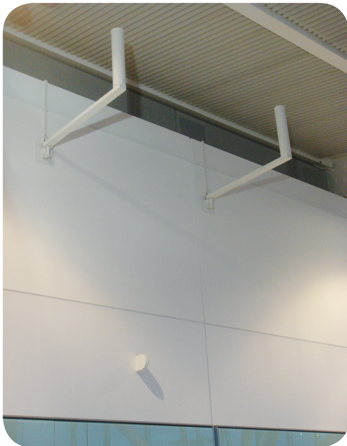
BDFPA-0.6-4.0-RL/1313 Ultra Wideband, Bi-Directional Antenna
