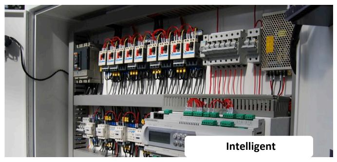
Advanced programmable controllers installed at Nanyang Technological University. Allow operators to have even greater accessibility and control over the chiller units.
