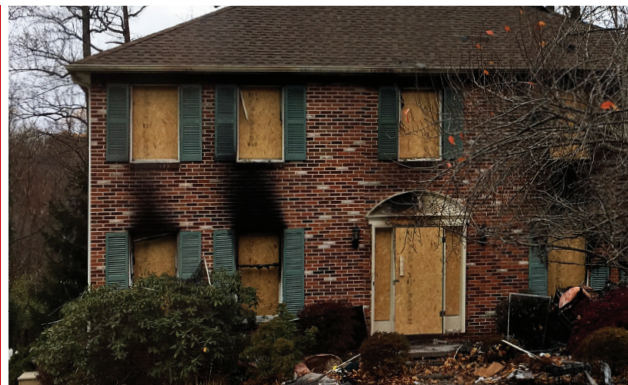
A failed MOV suppressor caused this 2016 NJ house fire.
