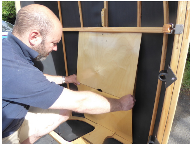
11. Positioning the two boards together, line them up as if they were hinged and push inwards to fit around the toggle as shown in fig 12.
