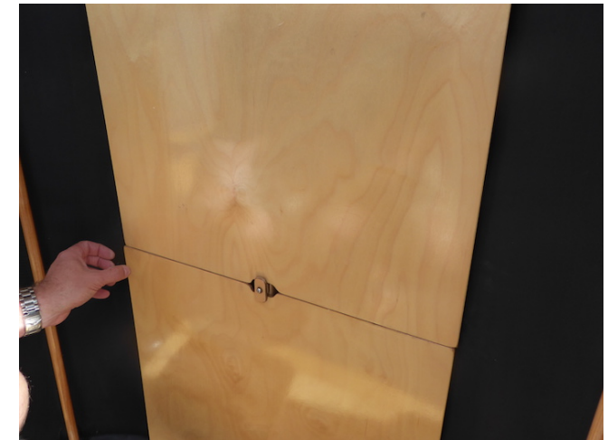
12. Floorboards are secured.
