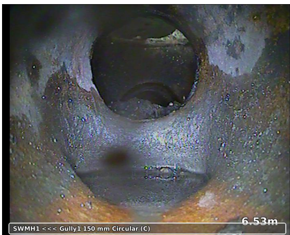
, 00:01:04, 6.53m Finish node type gully reference number: Gully1
