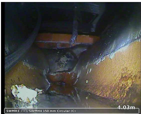
, 00:01:13, 4.03m Finish node type manhole reference number: SWMH4
