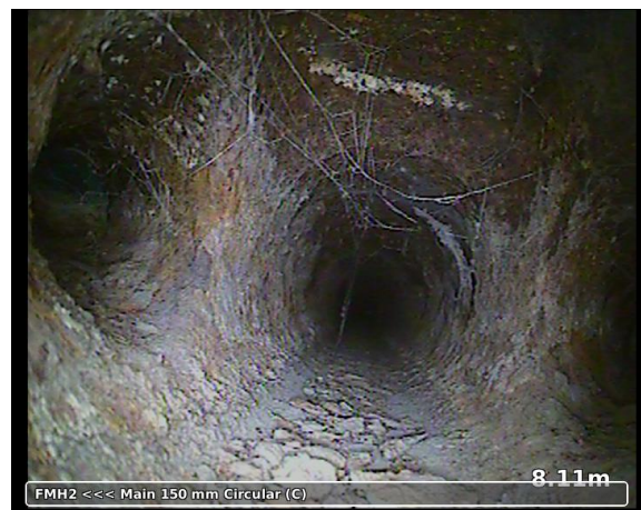
, 00:01:14, 8.11m General remark / enters hidden burns chamber
