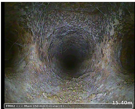
, 00:01:51, 15.40m General remark / Enters hidden burns chamber
