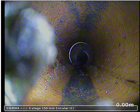
, 00:00:04, 0.00m Start node type manhole reference number: SWMH4
