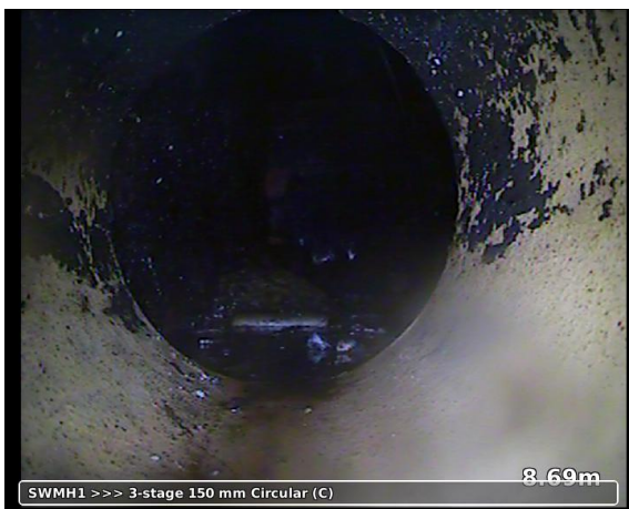
, 00:00:57, 8.69m Finish node type manhole reference number: 3-stage
