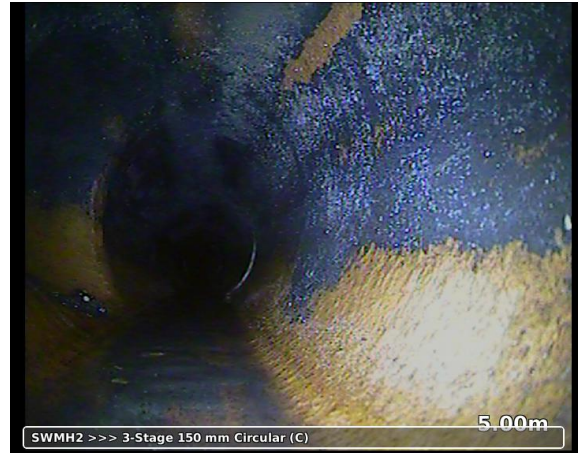
, 00:00:46, 5.00m Junction from/at 9 o'clock diameter: 150 mm / gully
