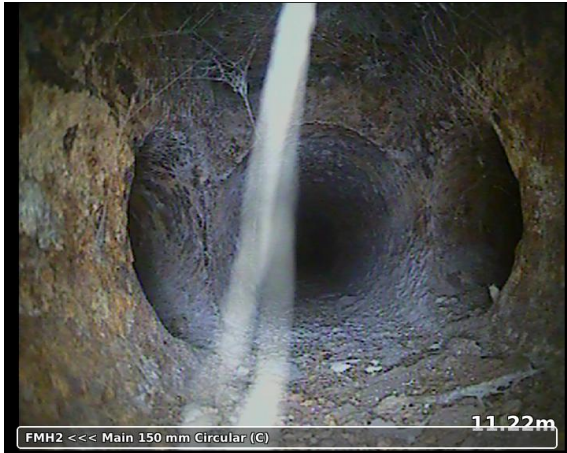
, 00:01:28, 11.22m General remark / Enters hidden burns chamber
