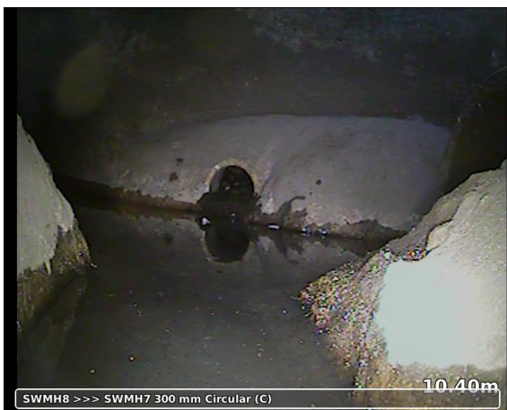
, 00:01:10, 10.40m Finish node type manhole reference number: SWMH7
