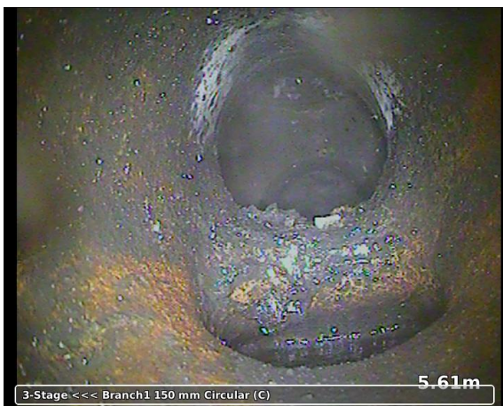
, 00:01:15, 5.61m Finish node type gully reference number: Branch1 / gully
