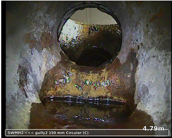
, 00:00:40, 4.79m Finish node type gully reference number: gully2
