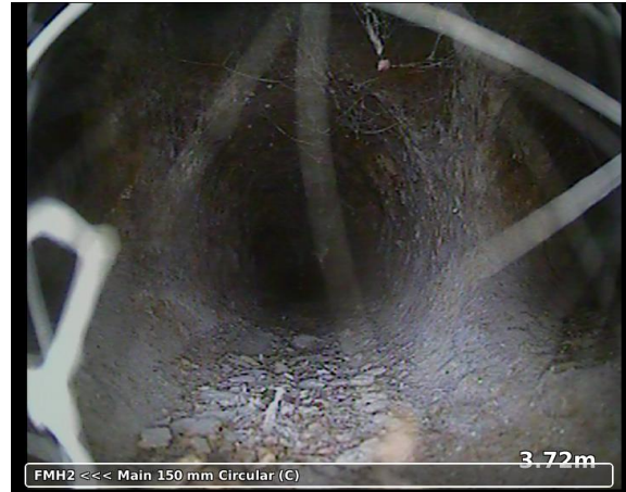
, 00:00:41, 3.72m General remark / Enters hidden burns chamber
