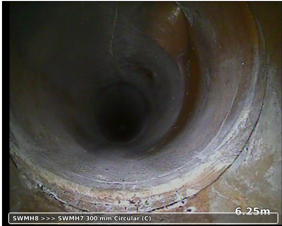
, 00:00:43, 6.25m Junction from/at 1 o'clock to 2 o'clock diameter: 100 mm
