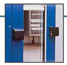
Dual photocells with reflector beams continuously scan opening for any obstruction. The door will return to fully open position if a beam is broken.
