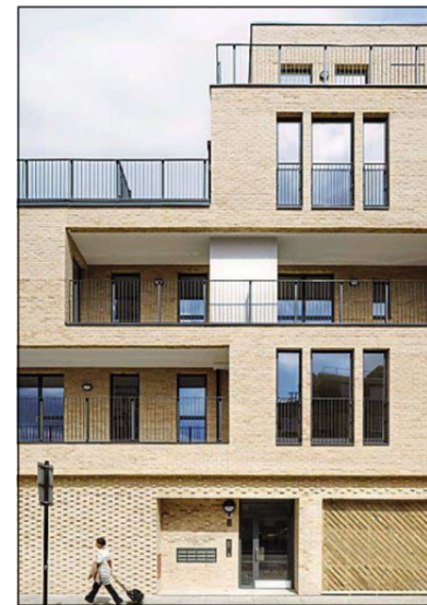
Small development category: above, creamy Ibstock bricks add grace and light at Elmwood Court, Battersea
