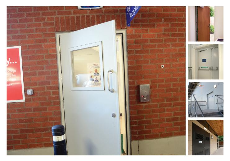
A resilient polyester powder-coat base primer on to a zinc-plated steel substrate reduces maintenance and improves the life of the finished coat. A factory-applied polyester top coat to most BS or RAL colours is available as an option.
