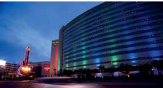
Roy Anderson Corp. built the Hard Rock Casino and Hotel in Biloxi, then rebuilt it after Hurricane Katrina in 2005.
