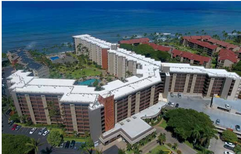
CRW reroofed the Aston Kaanapali Shores on Maui.
