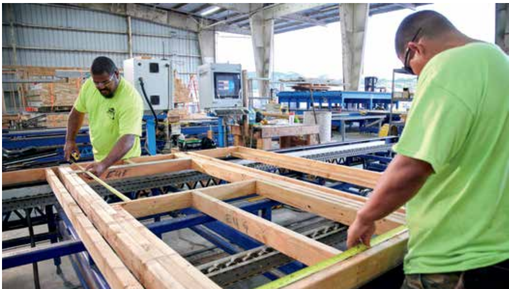
HPM wall panels under construction.
