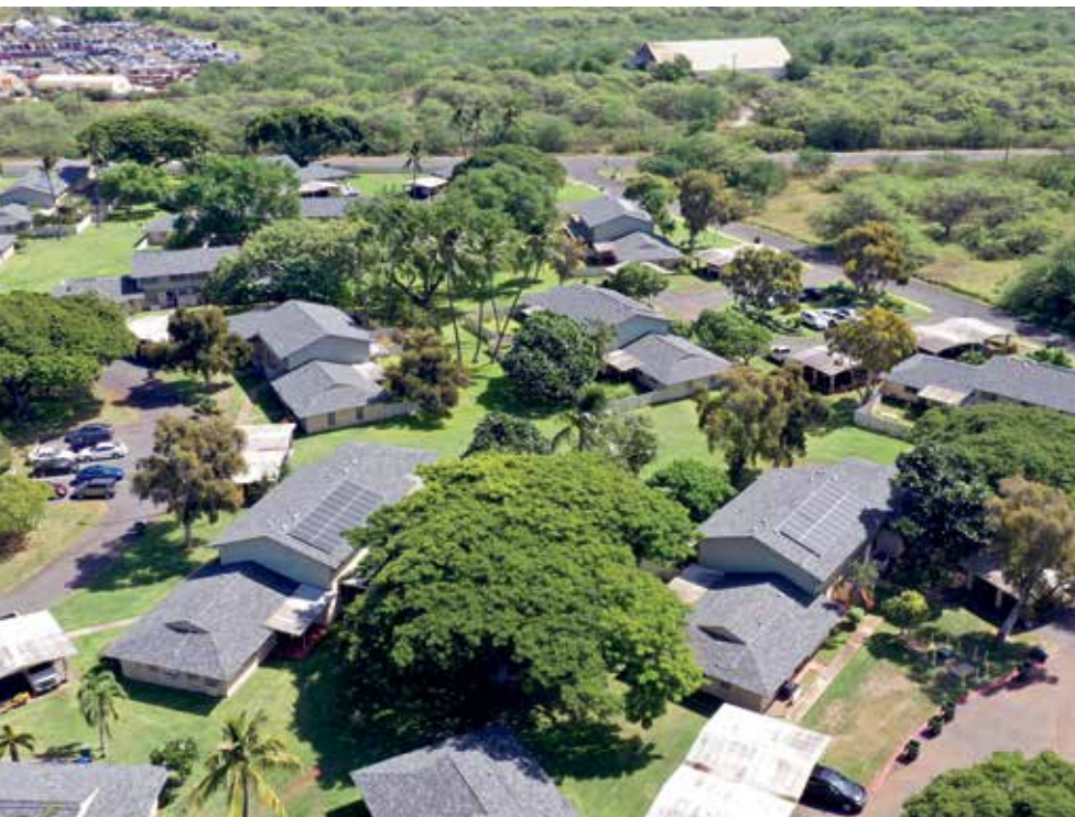
Tory's Roofing's jobs last year included a residential area of Kalaeloa.
