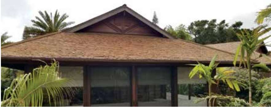
A Beachside Roofing project: Four Seasons Koele Spas
