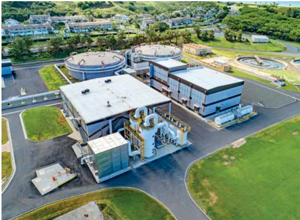
Kailua Regional Wastewater Treatment Plant
