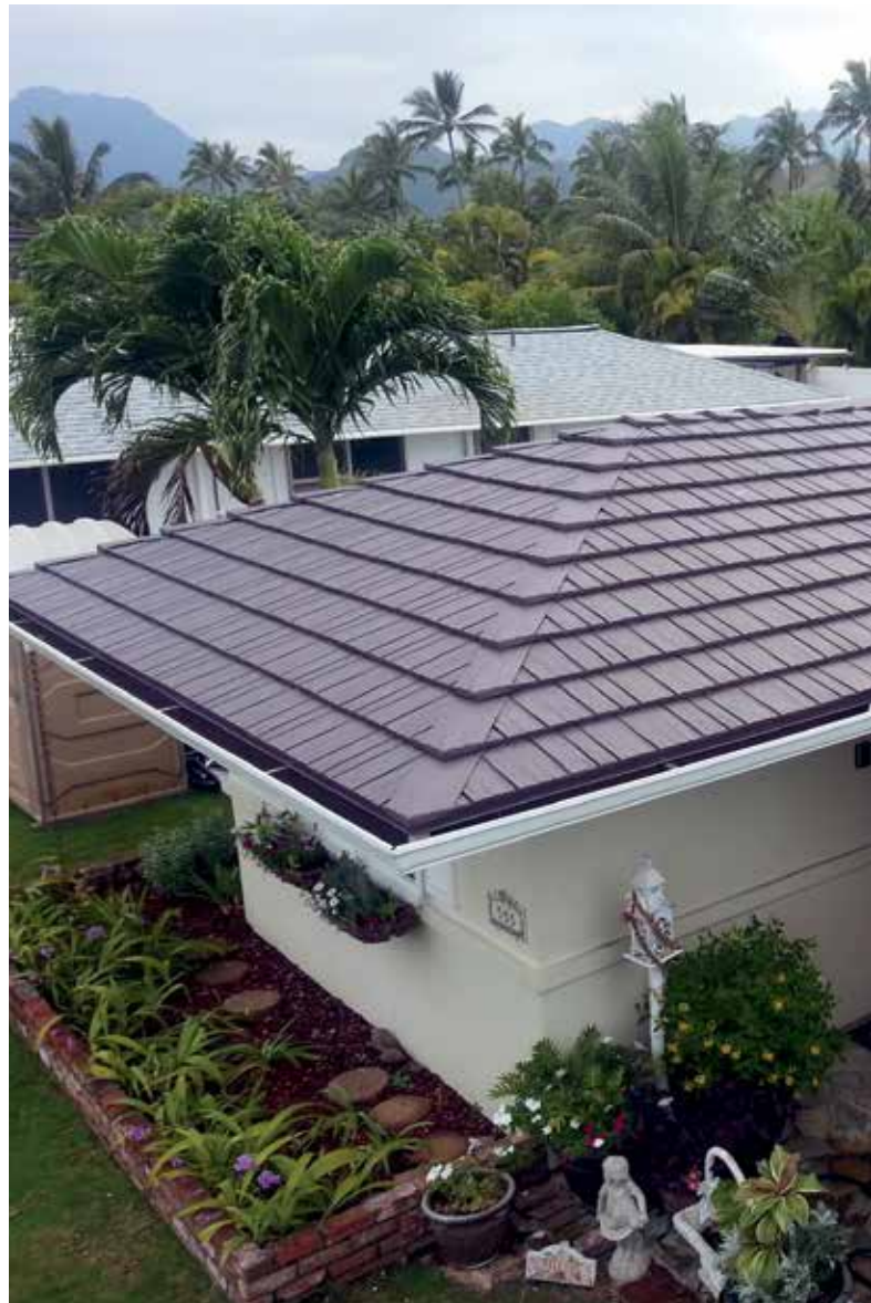
David's Custom Roofing & Painting installed many residential roofs in 2018.
