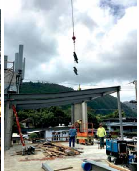
Framing up the new bank
