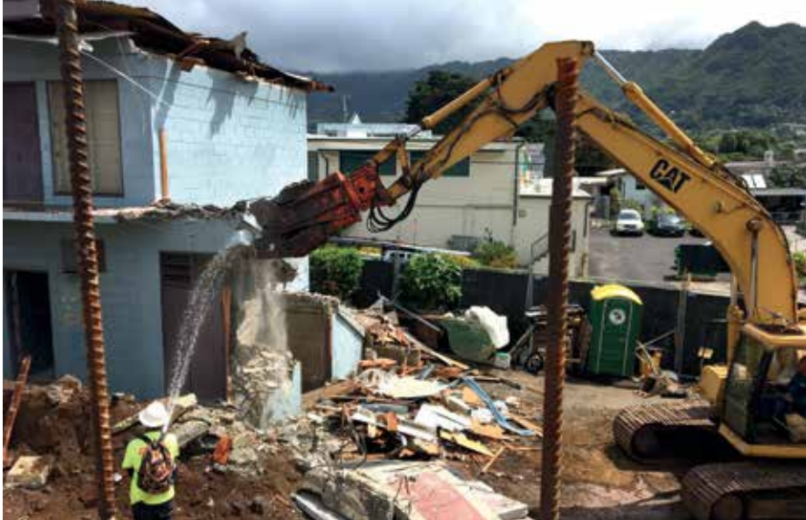
RSI demolished an existing structure at the Manoa site.
