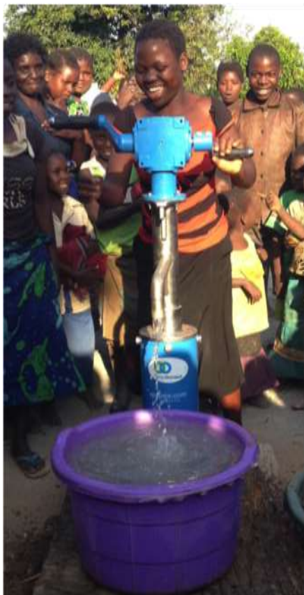
Figure 9. The first LifePump in Malawi was installed November 2013. The borehole was too deep for an Afridev and was declared dry until the LifePump arrived and could reach the water.
