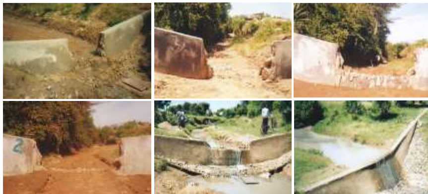
Figure 2: A sand storage dam was raised 3m in 6 stages of 0.50 m in one rainy season, in Kenya. Source: (Nissen-Petersen, 2006).
