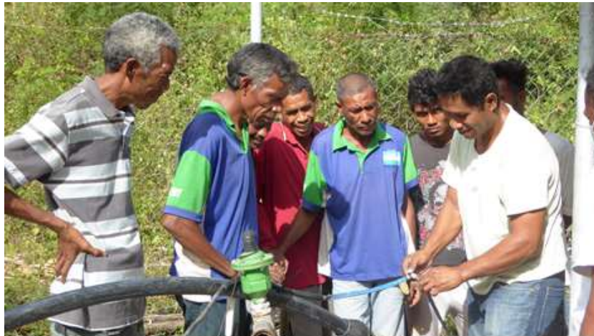
Figure 3-40: BESIK pump technician installing a new pump at Rau Moko in Lautem municipality (BESIK, 2015)
