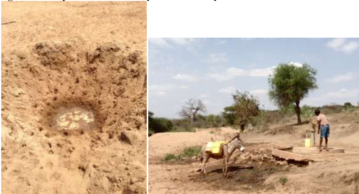
Figure 3: Abstraction From a Wide Bore Shallow Well. The donkey is standing on the sand dam surface.
