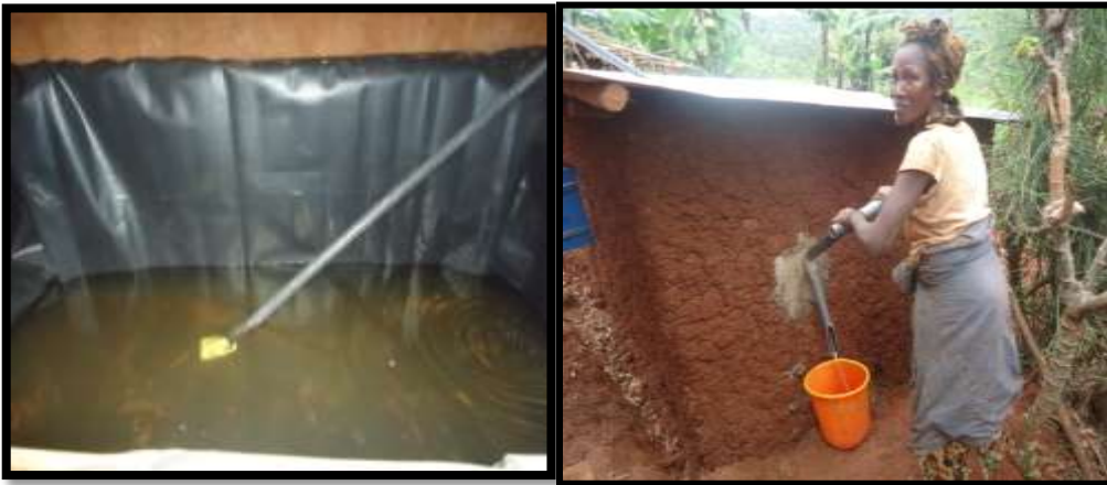
Photo 1: Semi under-ground tank technology, Nyanza District.
