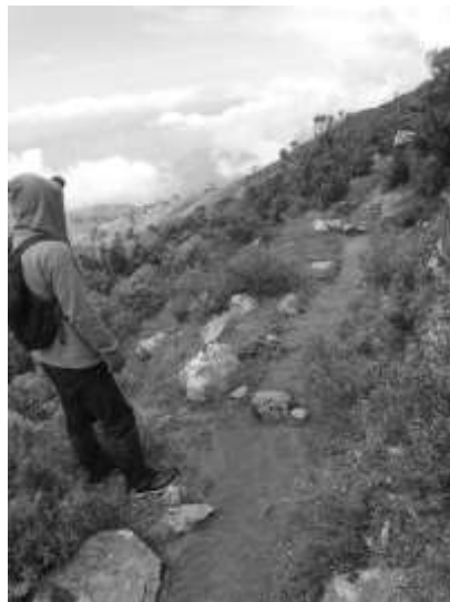
Fig. 9 - The end of a feeder canal in Tupicocha
