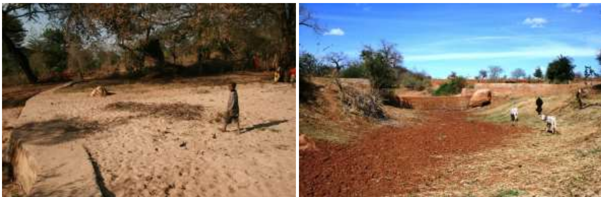
Figure 1: A successful small-scale sand storage dam (left) and a silted-up reservoir (right), in Kenya.
