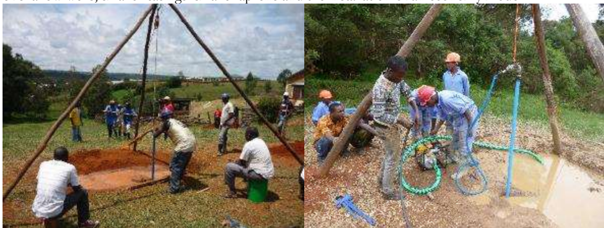
Drilling a tube well of 30 meters deep with the SHIPO drill method The SHIPO drill combined with jetting
