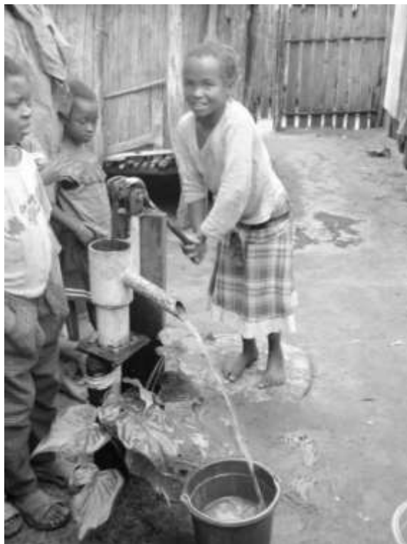
Figure 1: (a) Pitcher Pump in use in Tamatave, Madagascar [left] (Photo: M. MacCarthy); (b) Diagram of Pitcher Pump system [right] (Source: Artwork by Linda Phillips. Reproduced from Mihelcic et al. (2009); with permission from ASCE.)
