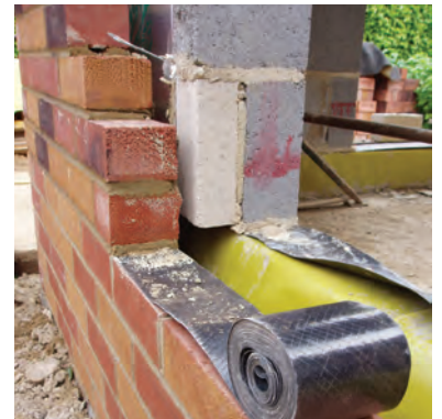
Damp course membrane joining
