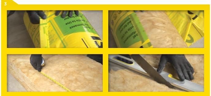
Slit the packaging on the cut section of the roll to allow the Metac to unroll and allow full thickness recovery. Measure and cut the roll to the required length with a straight edge and a sharp insulation knife.
