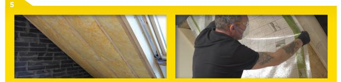
Once the rafters are filled with Metac, apply a vapour control layer (VCL) to the underside of the rafters, following the manufacturer's instructions and recommendations.
