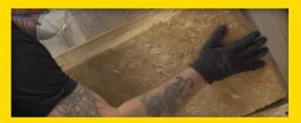
Finally, a thermal laminate, insulation with plasterboard or another layer of Metac can be installed between 50mm counter battens fixed at 600mm centres.
