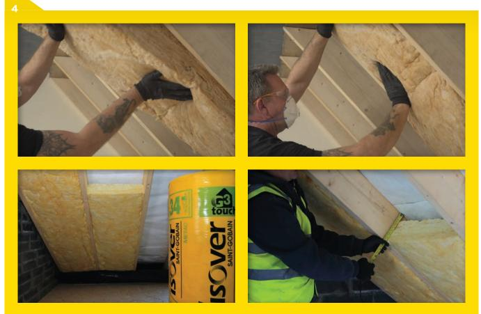
Push and friction-fit the Metac between the rafters working from the bottom up, keeping the lower face of the Metac flush with the rafters. Ensure ventilation voids are maintained where required.
