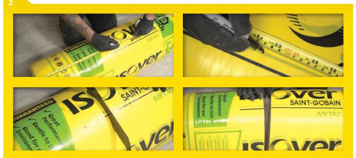
Measure and cut the roll with an insulation saw or insulation knife to fit the horizontal width of the gap between the rafters whilst still in its packaging – adding an extra 10mm width to the Metac to allow for a snug fit.
