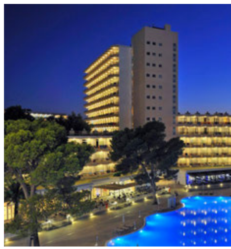
HOTEL MELIA SOL BARBADOS | Mallorca, Spain Rooftop units KCR , Chillers KWE & Fan coil units
