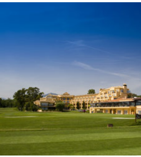
HOTEL GUADALMINA | Marbella, Spain Chillers KWA with full heat reclaim
