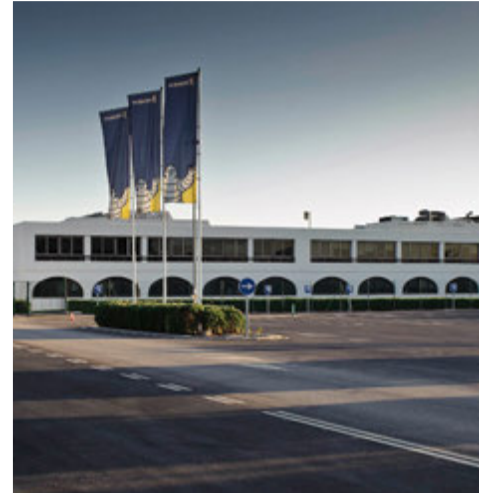
MICHELIN EXPERIENCE CENTRE | Almería, Spain. Rooftop units KCR
