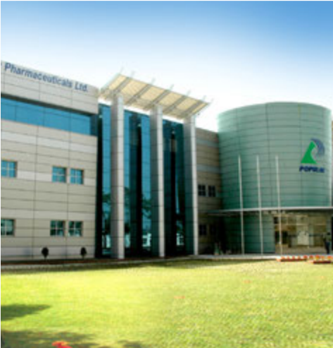
POPULAR PHARMA | Gazipur, Bangladesh Chillers KWE and AHUs KTS
