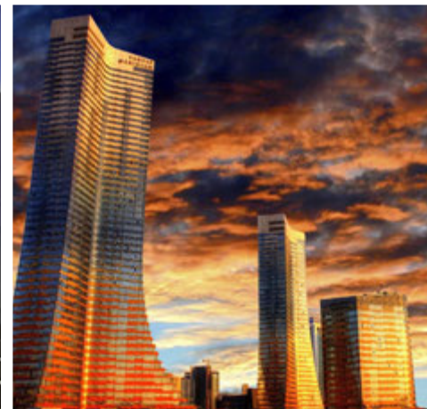
VARYAP MERIDIAN | Istanbul, Turkey Chiller KWB
