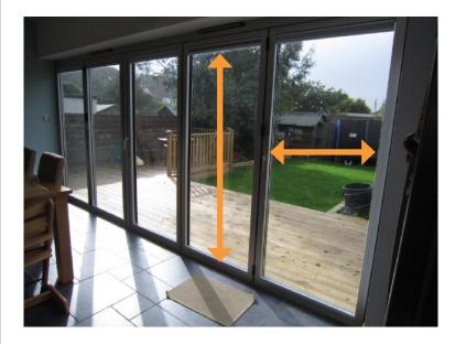
When an order is placed you must deduct 4mm from the width to allow for clearance and 10mm from the drop of the blind to add tension to the blind.
