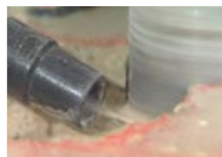
Vacuum drilling slurry
