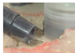
Vacuum drilling slurry
